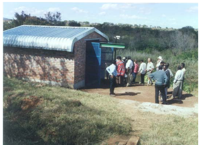
Figure 2: Commissioning a new irrigation system. This is an essential component of project implementation.
